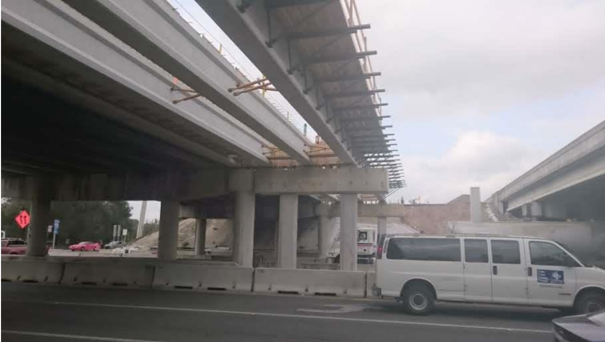
Temporary Beam Bracing and Deck Forming
