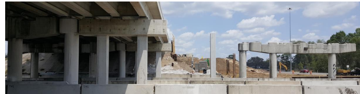
Bridge Widening and Temporary Shoring Support
