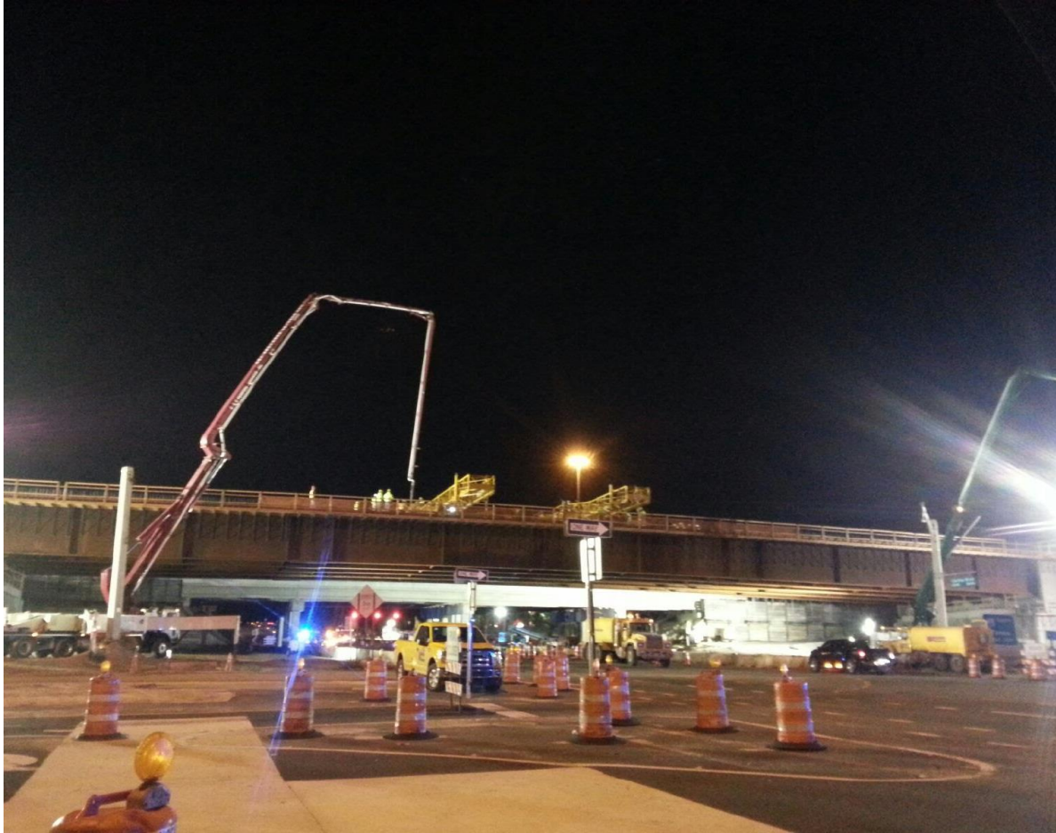
NB Bridge Deck Pour In One Single Night Operation With Two Terex® Bid-wells
