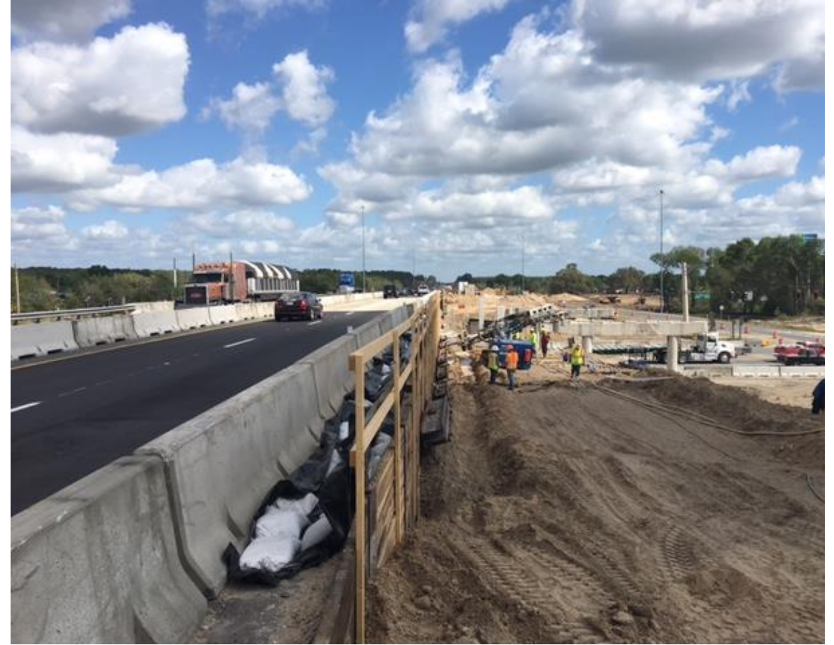
Soldier Pile and Lagging Wall with Prestressed Soil Anchors
