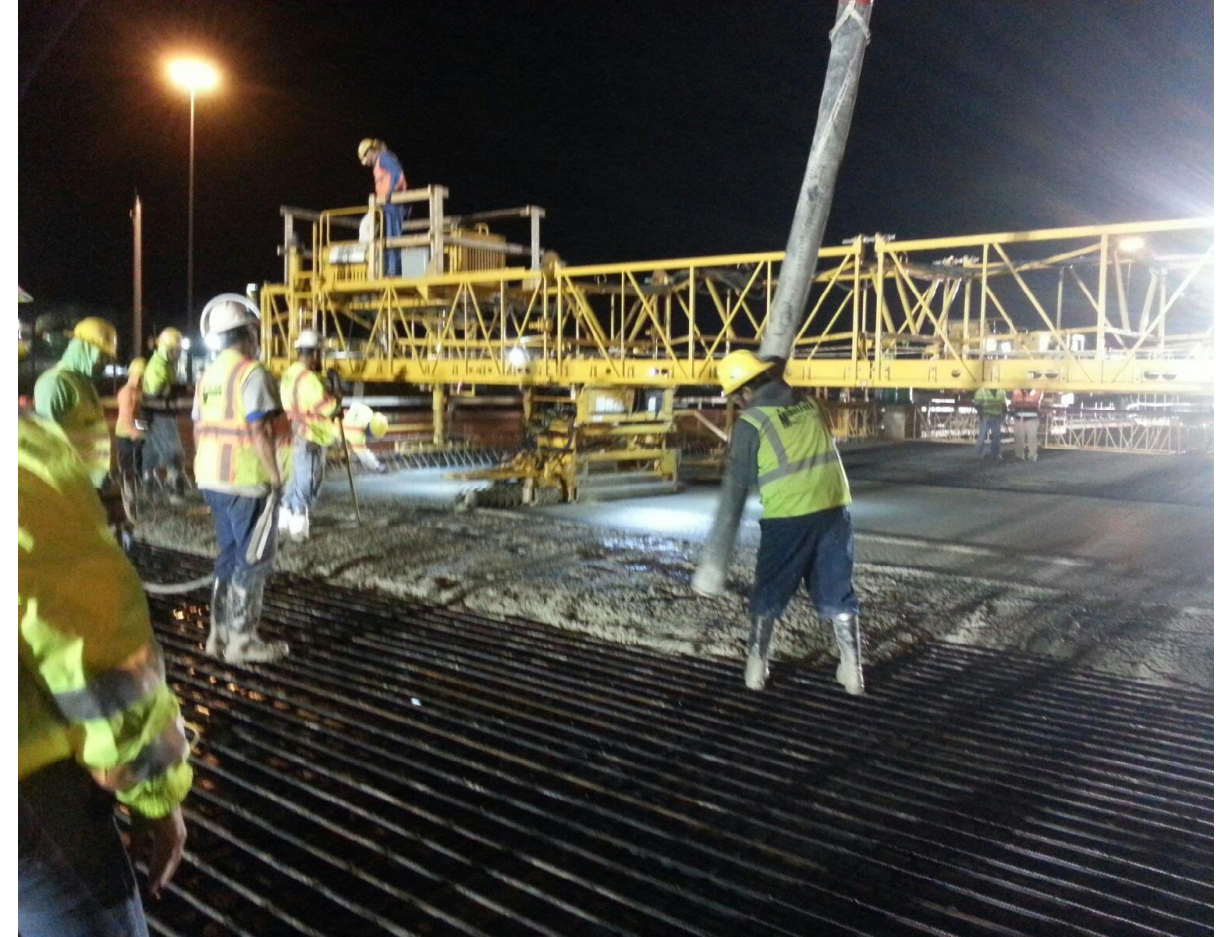
NB Bridge Deck Pour In One Single Night Operation With Two Terex® Bid-wells
