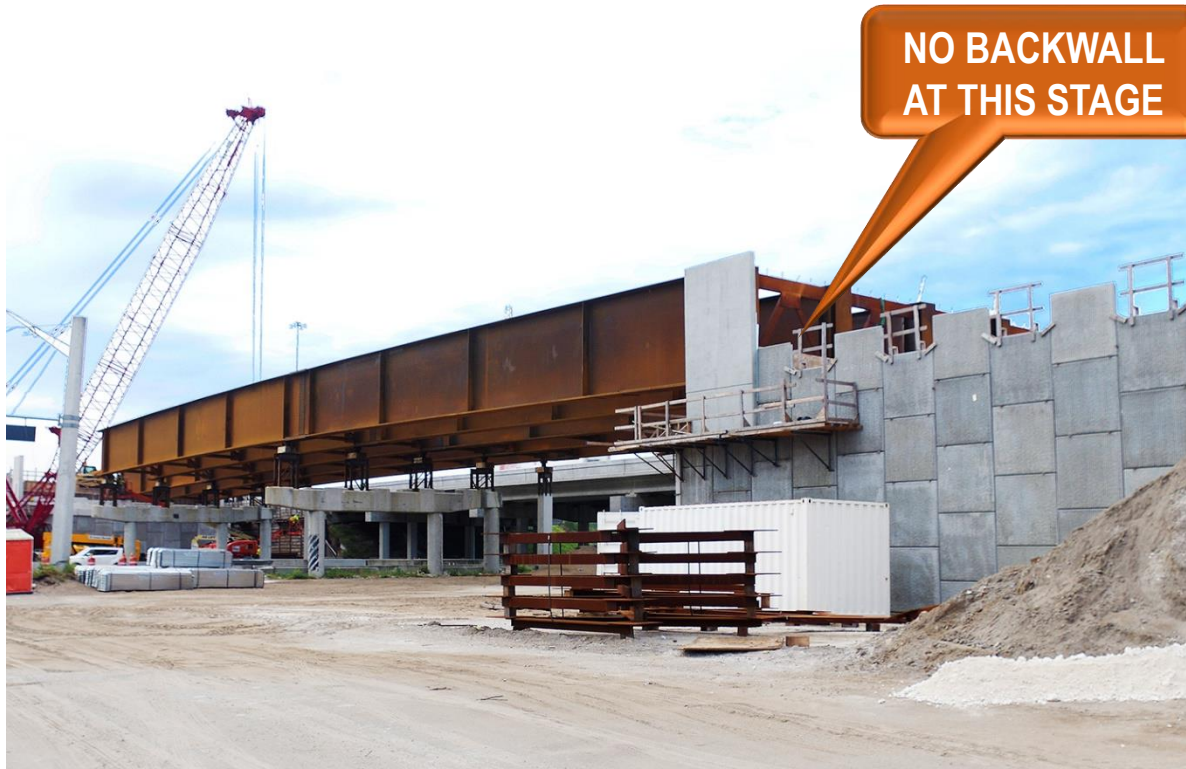
NB Bridge Steel Girder Segments 2 and 3 Erection
