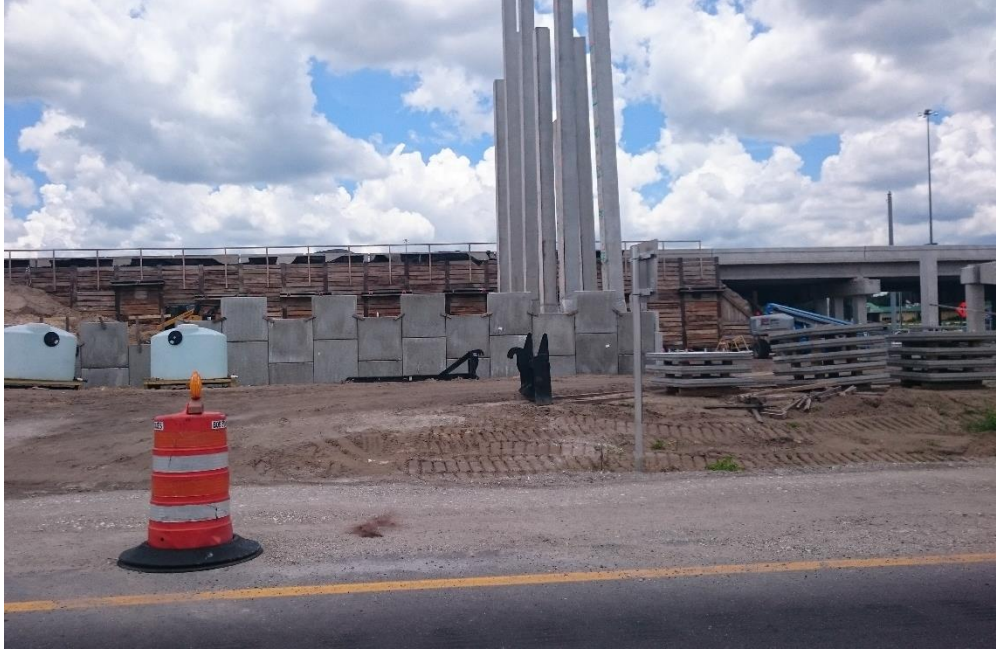
Foundations and Wall Construction
