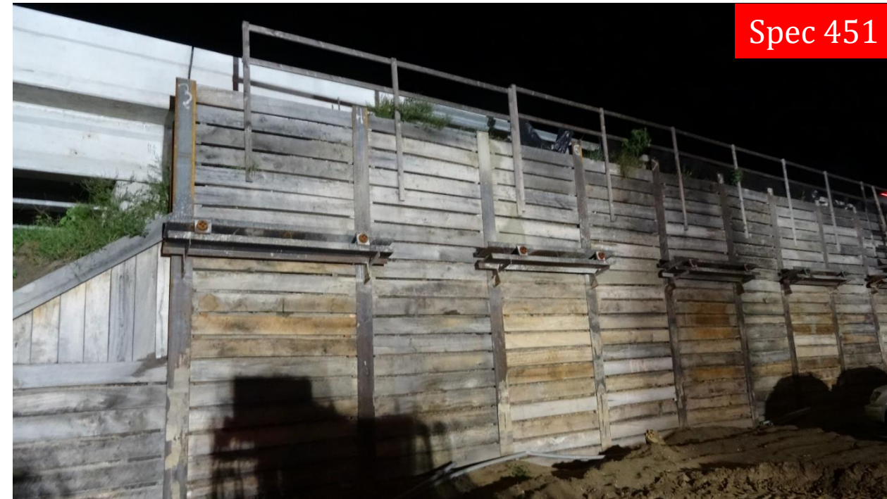
Soldier Pile and Lagging Wall With Prestressed Soil Anchors
