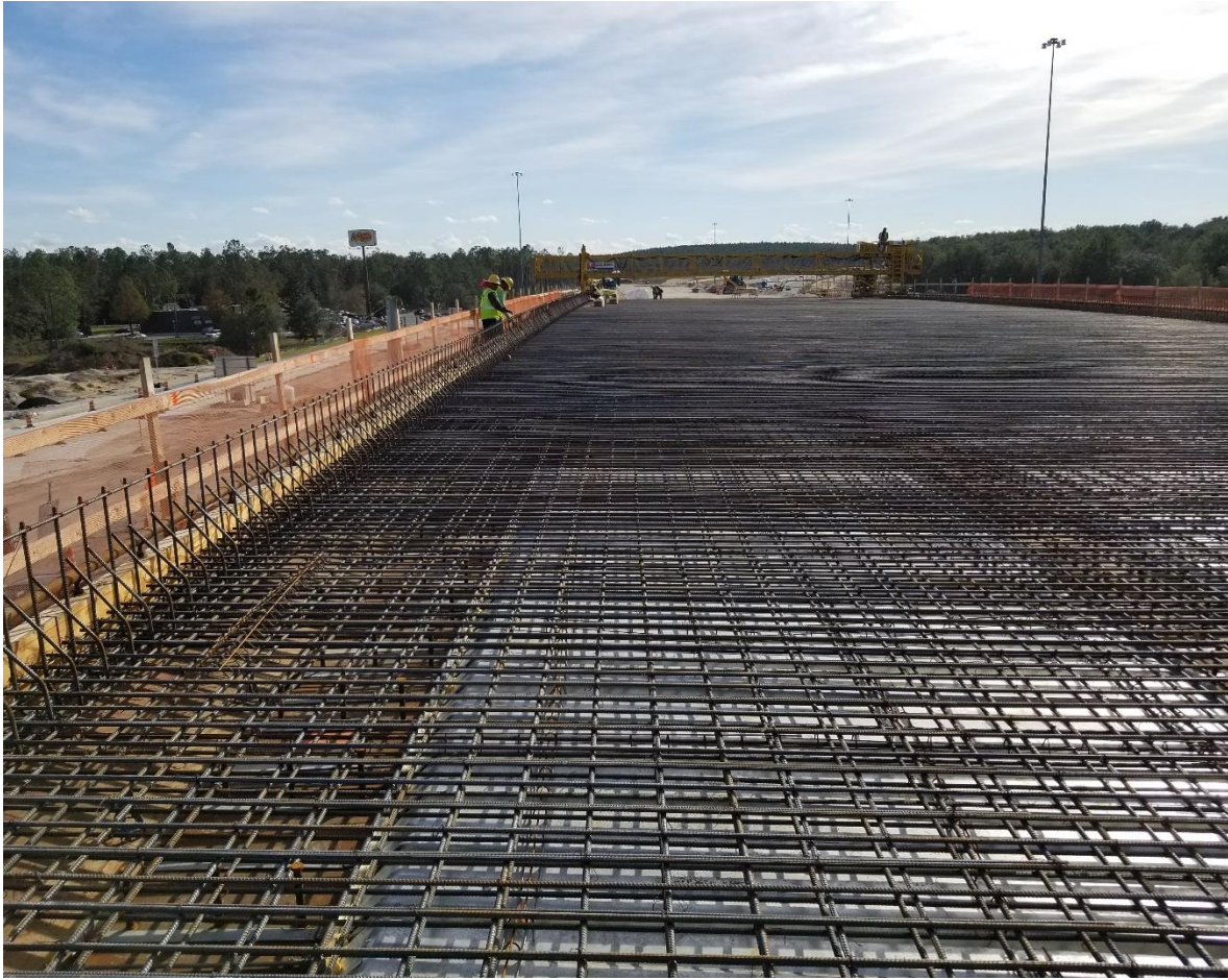
Preparing For Deck Pour and Setting Up Terex® Bid-wells
