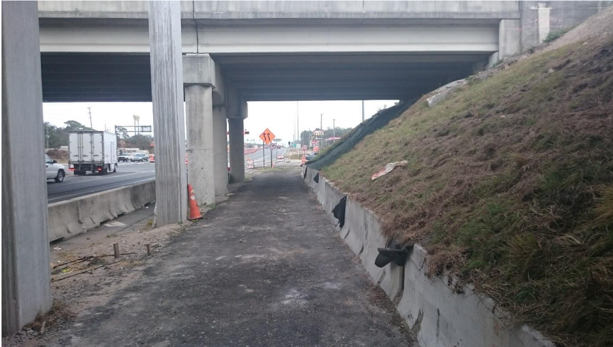
Temporary Shared Path and Slope Protection
