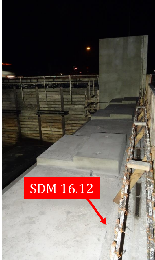
End Bent With Trough For Water and Weathering Iron Oxide Runoff (Backwall Not Poured)
