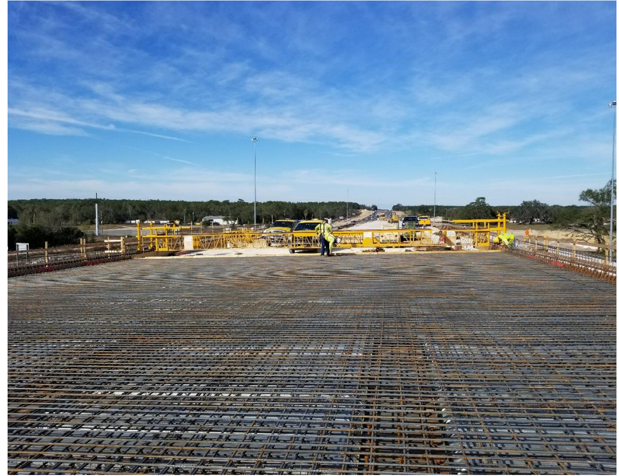
Preparing For Deck Pour and Setting Up Terex® Bid-wells
