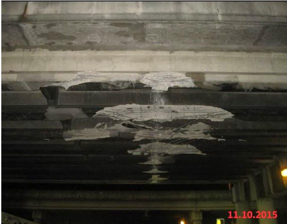
NB Bridge Beams Damaged By Truck Impact
