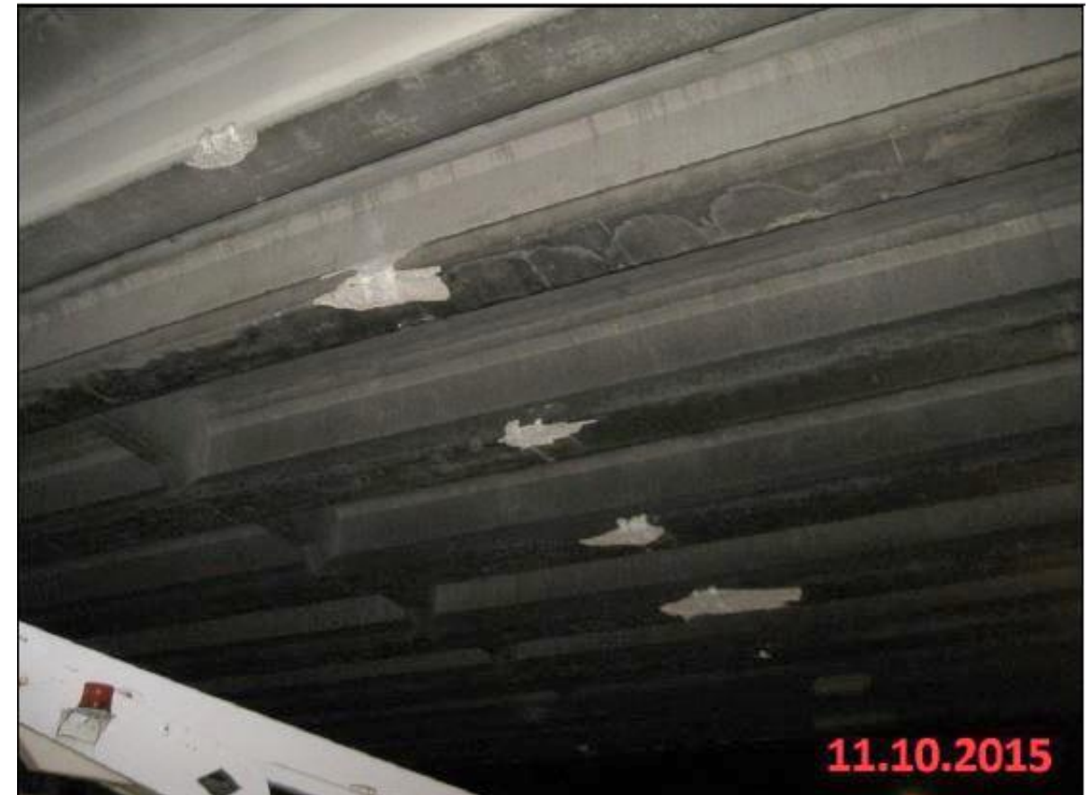
SB Bridge Beams Damaged By Truck Impact
