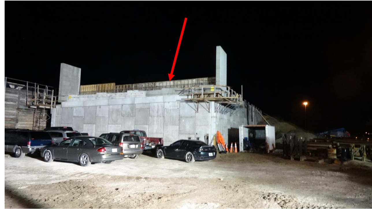
End Bent Cap, Wrap Around MSE Retaining Wall and Pressure Relief Wall (Backwall Not Poured)
