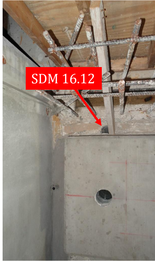
End Bent With Trough For Water and Weathering Iron Oxide Runoff (Backwall Not Poured)
