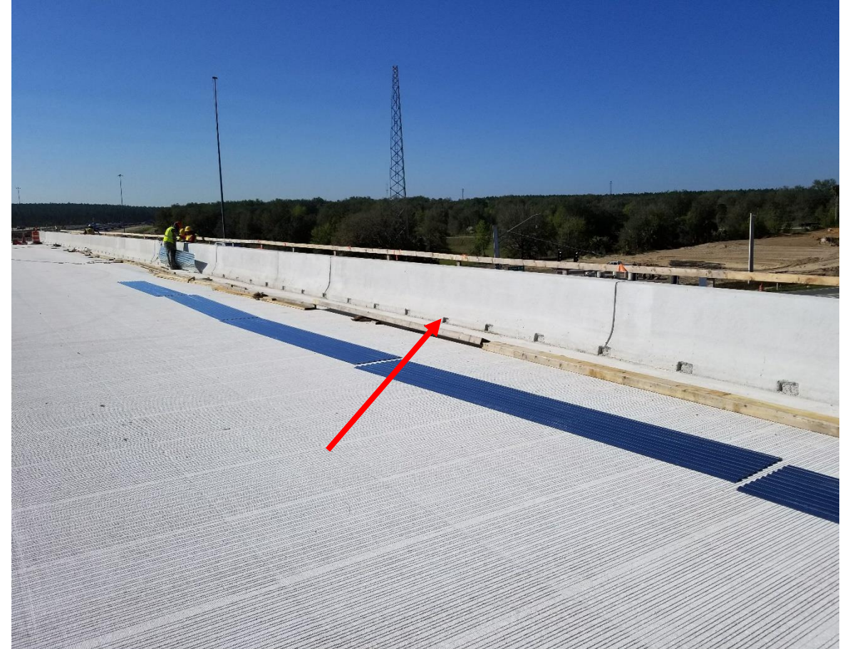
Railing Slots For Temporary NB Bridge Drainage System
