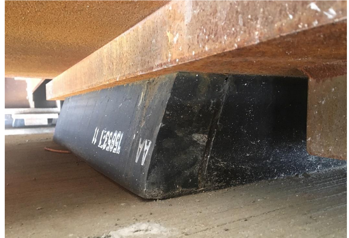
Bearing Pad Shear Deformation After Deck Pour and Prior to Re-setting
