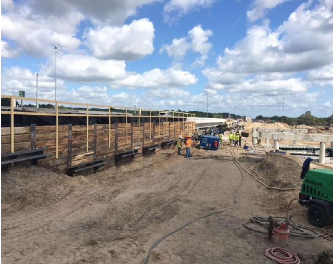
Soldier Pile and Lagging Wall with Prestressed Soil Anchors
