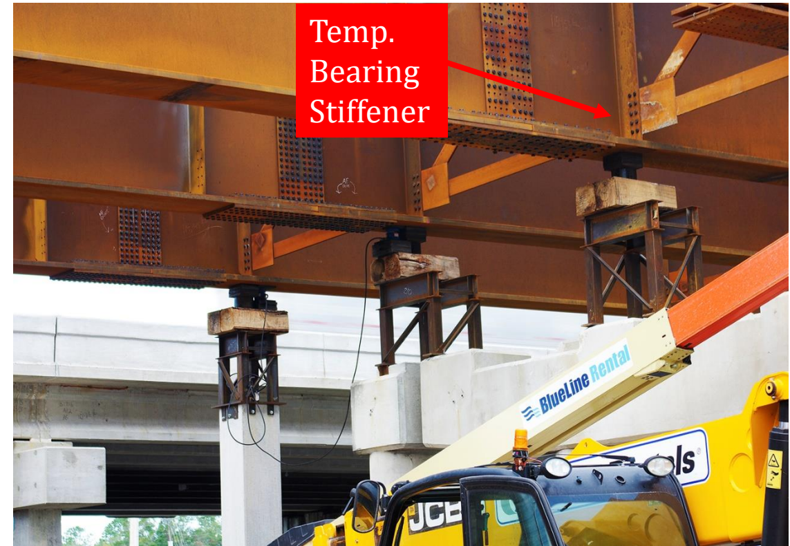
Temporary Shoring Support For NB Bridge Steel Girder Erection
