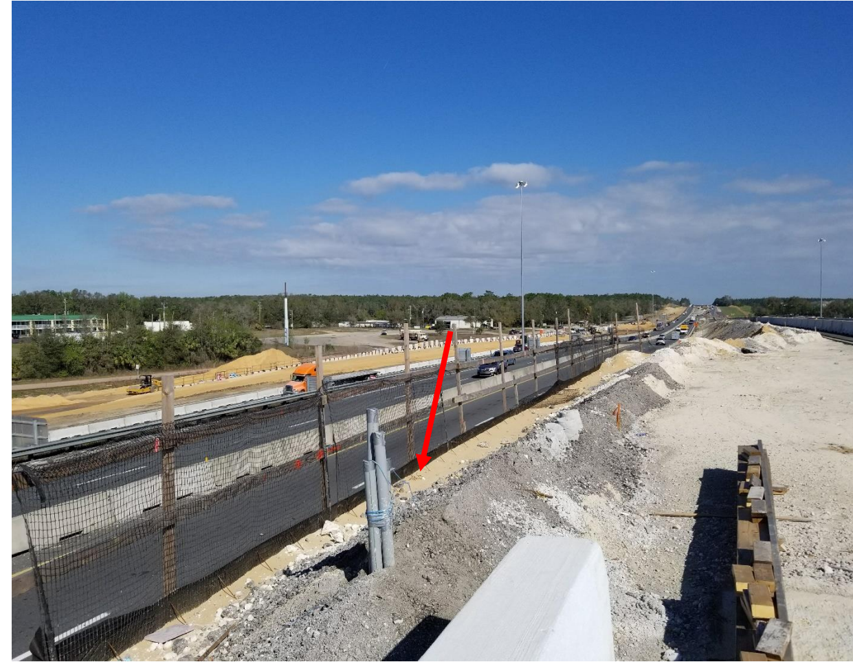
Phase 2 Temporary Critical Walls
