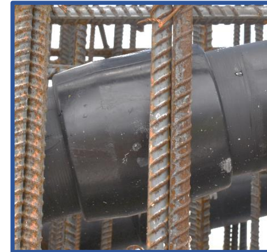
HDPE Pipe with Electrofusion Coupler
