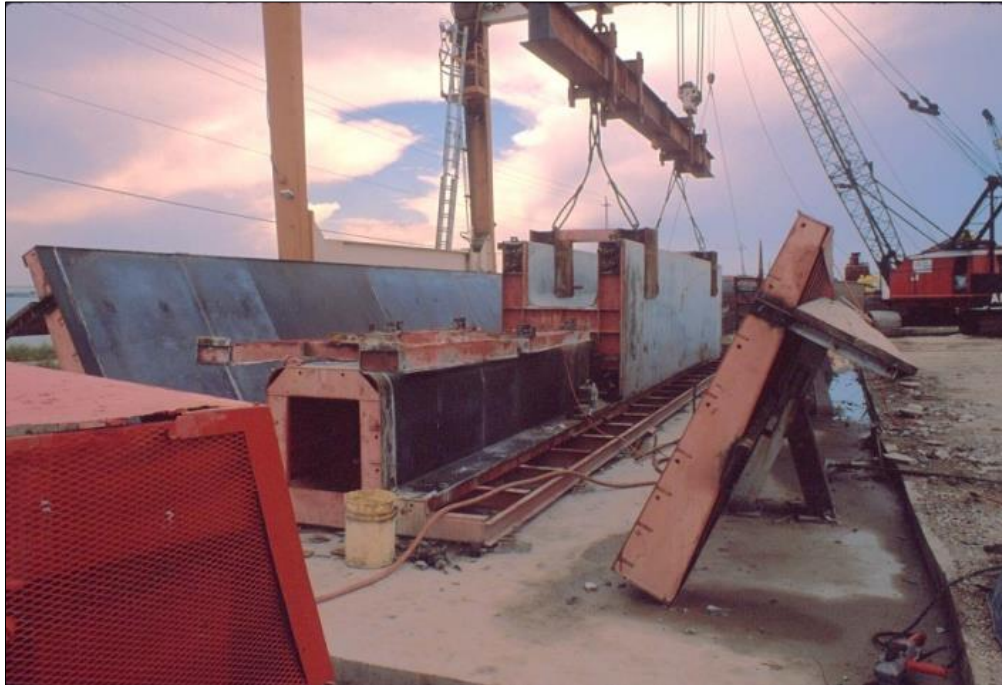
View of precast column segment formwork in the precasting yard.
