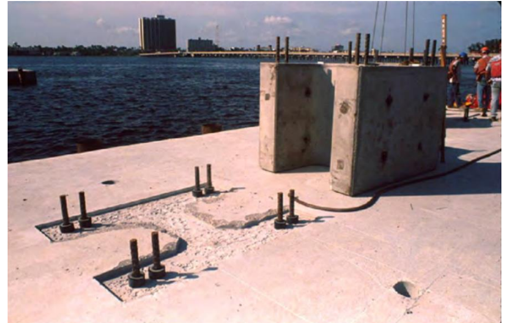
View of precast column segment being set on CIP footing.
