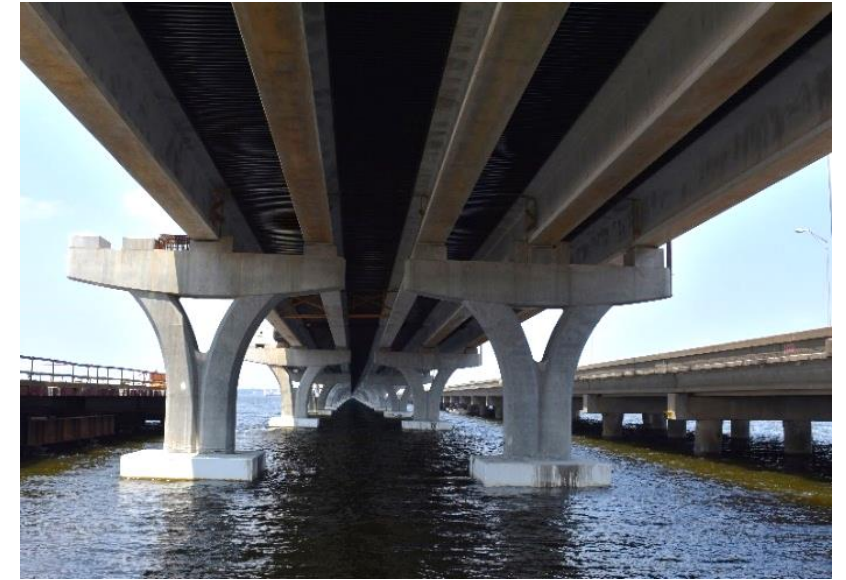
View of low-level precast piers supporting vehicular bridge over Pensacola Bay.
