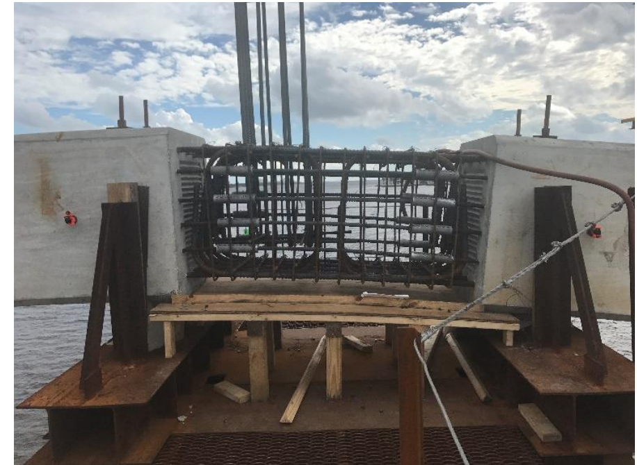
Visual rendering of arch rib precast section closure pour detail (Acknowledgement: WSP).
