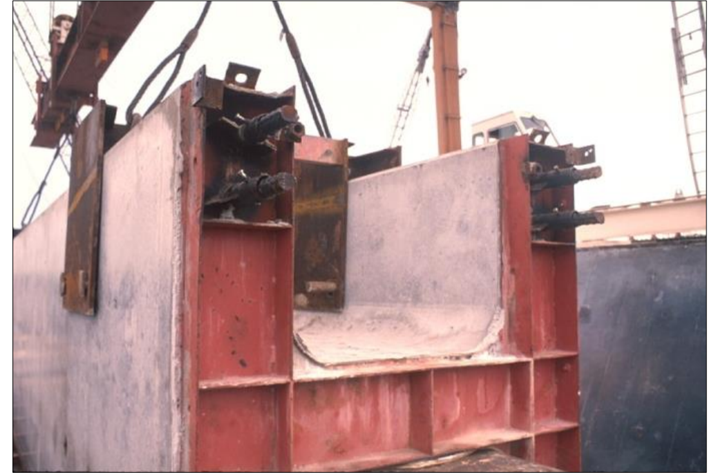
View of precast column segment with bulkhead form.
