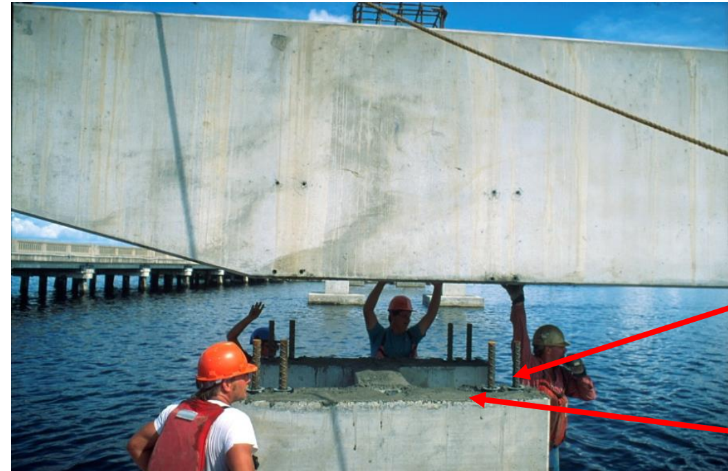
Erection of precast cap assembly during construction.
