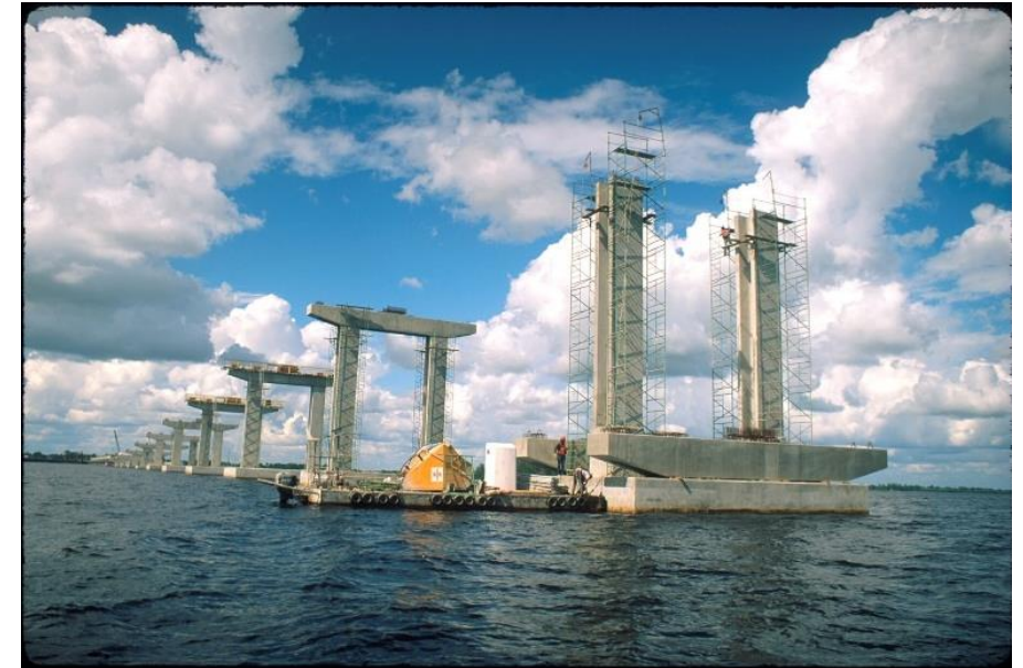
Top: Overall view of precast pier construction for the Edison Bridge.
