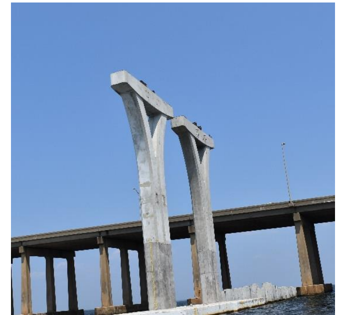
View of completed high-level pier assembly.
