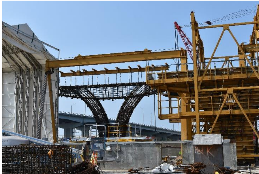
View of low-level precast pier assembly in the precast yard.
