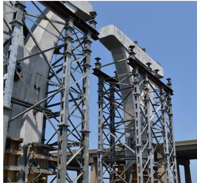
View of high-level precast pier assembly on falsework.
