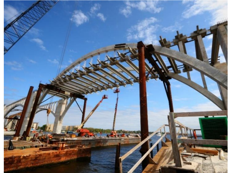
View of Veterans Memorial Bridge main span construction.
