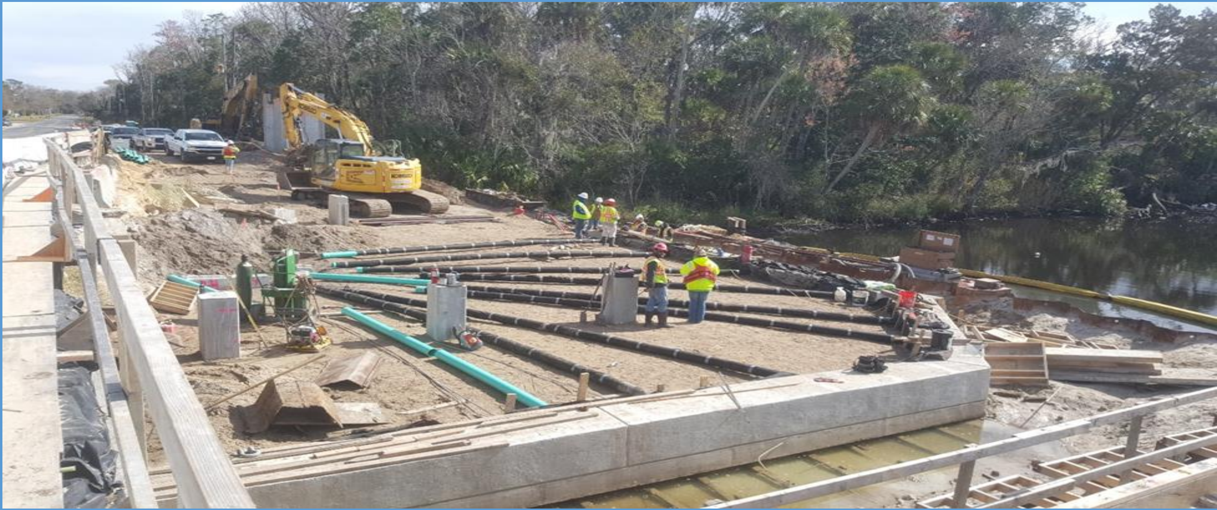
Deadman and Anchor Seawall
